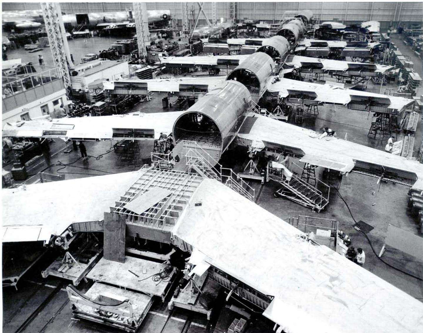
ABOVE: The 'joining line' at Boeing's Renton plant, where wings and centre fuselages came together. This early photo shows the first production 707s with the second aircraft for Pan Am at the top. In the bay to the left is the final assembly area for KC-135s. Boeing via the Aviation Picture Library
