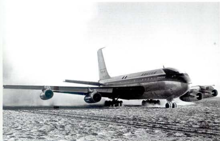
BELOW AND RIGHT: As part of tests for the very large aircraft (later C-5) programme, a double-wheel undercarriage was installed on the Dash 80 and many take-offs and landings were made on the Harper Dry Lake, California in 1959. The temporary landing gear was not retractable. Boeing via the Aviation Picture Library
